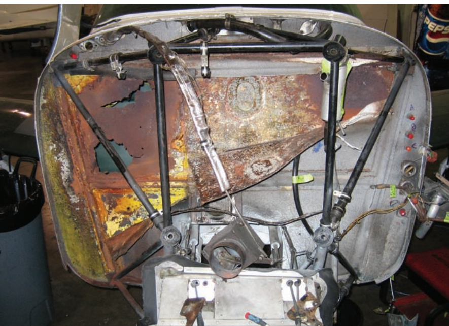
Firewall corrosion damage discovered on a 1978 Piper Lance.
